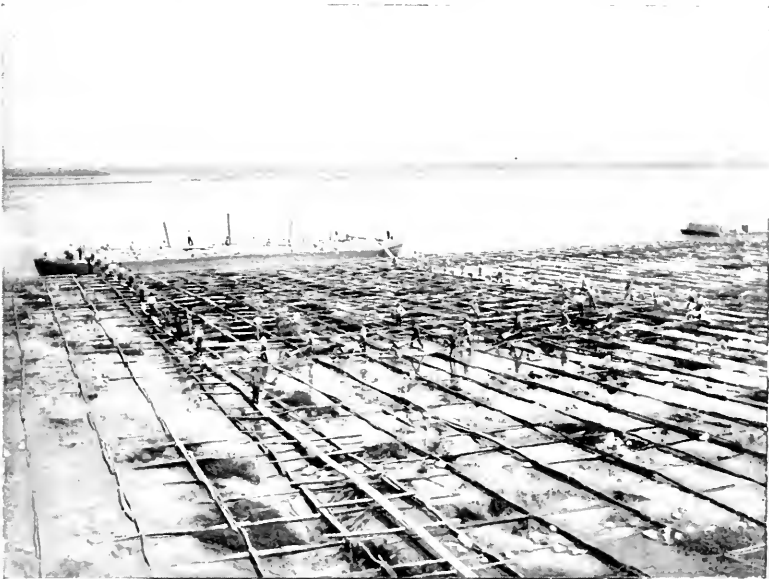
BALLASTING WOVEN MAT PRIOR TO SINKING.
